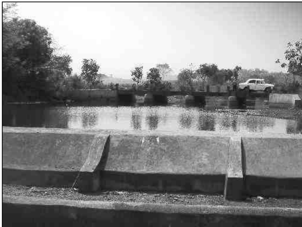
Figure No-4: Check Dams / Nala bunds at Jogta Nala, near Nischitpur OCP Mine, BCCL. This Recharge structure is within the buffer zone (1.8 km towards east of Cluster-IV).
