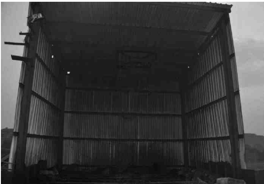
Water Arrangement at CHP Hooper
